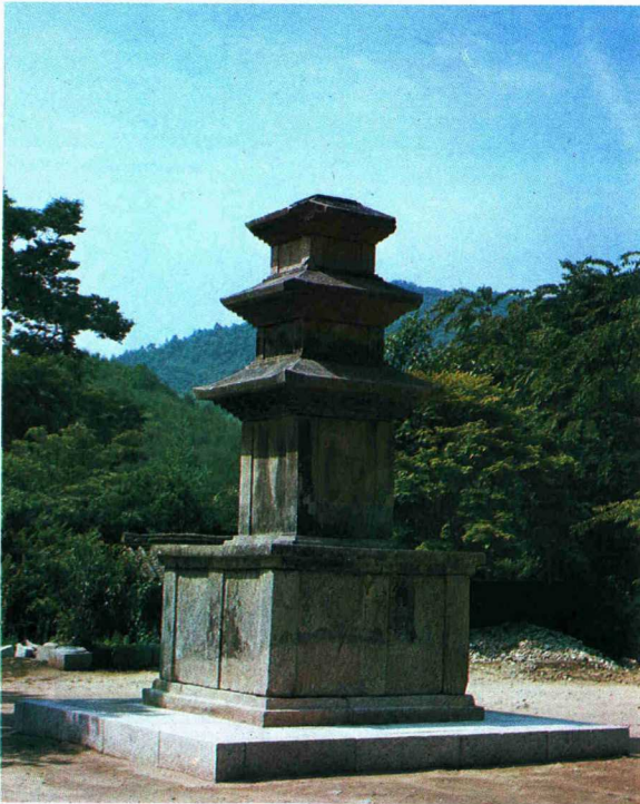
A three-story stone stupa
